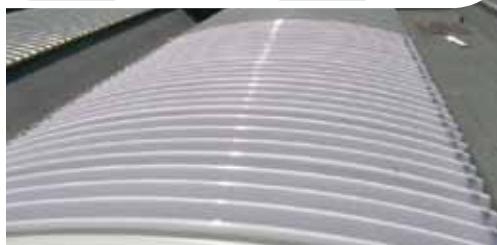
**arcoplus®1000** and **SUPER1000** are modular systems with corrugated PC sheets UV protected used to create flat or curved roofing, translucent curtain walls and skylight. They can be used in continuous applications or with other insulated corrugated panels.
